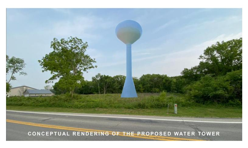
This project will erect a 150,000-gallon elevated water storage tank at a site along East Bayshore Road, on the north side of the road across from Bradley Lane.
