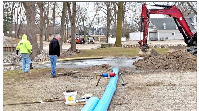
At Bay Point, looking north. 8-inch water main pipe being pulled under the waterway, 12/22/22
