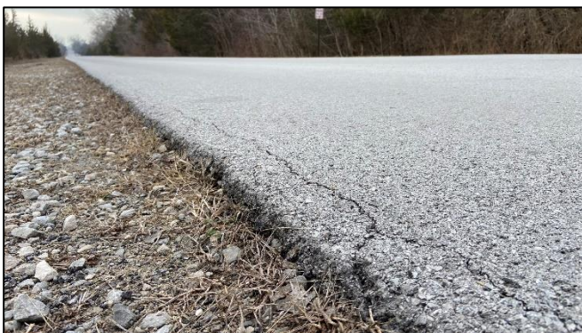
Alexander Pike's pavement showing pitting due to loss of the fines. Rejuvenator helps to reduce the rate of loss.
