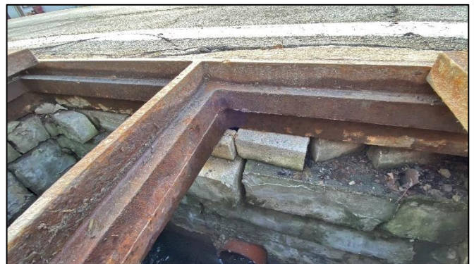
Grate frame w/ loose bricks, 233 E Main, 1/9/23
