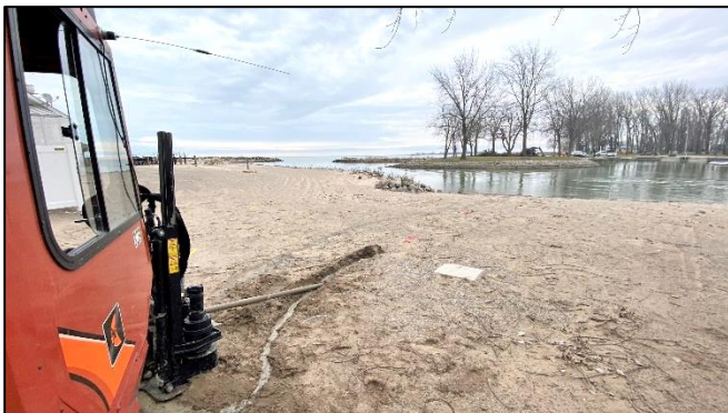
Looking south. Directional boring equipment pulling the 8-inch water main pipe under the waterway, 12/22/22
