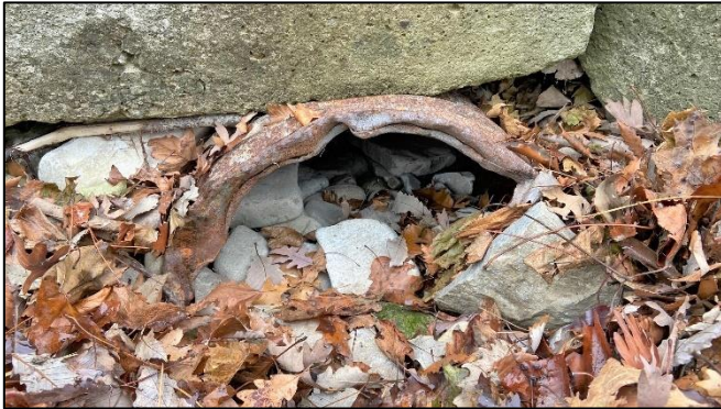
Storm drain outfall pipe mostly plugged, 1/5/23
