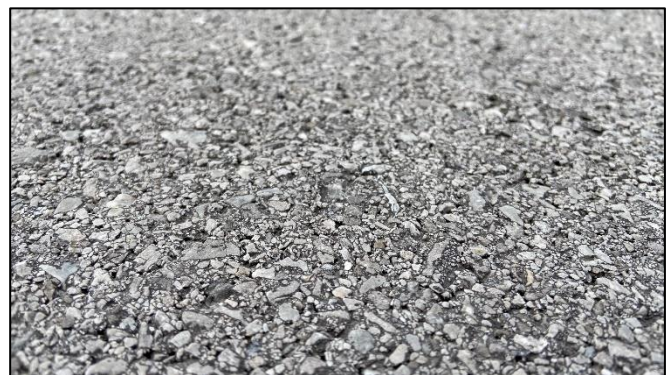
Alexander Pike's pavement showing pitting due to loss of the fines. Rejuvenator helps to reduce the rate of loss.
