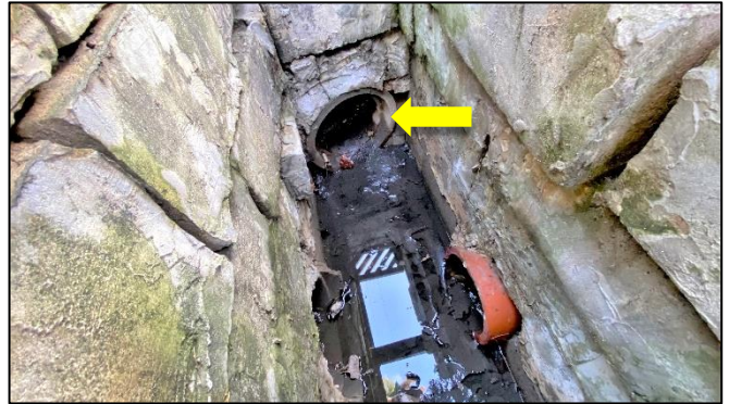
Catch basin, 10-inch outlet pipe filled with sediment
