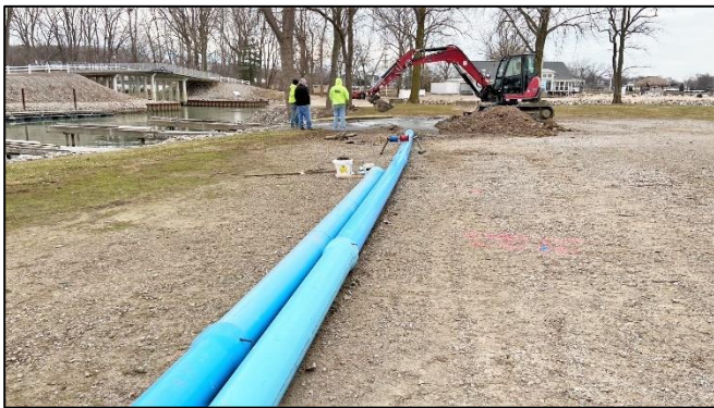
At Bay Point, looking north. 8-inch water main pipe being pulled under the waterway, 12/22/22
