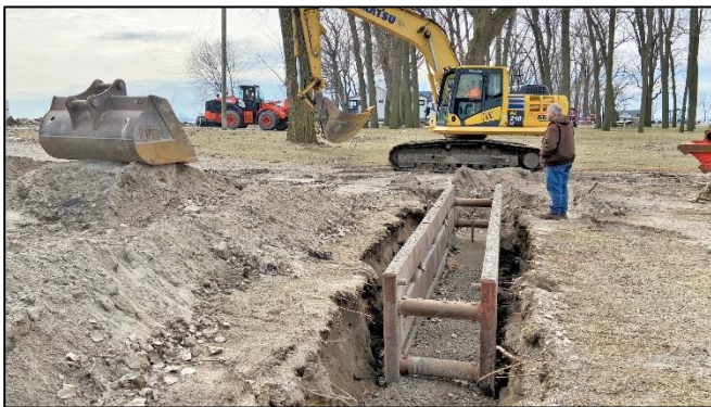
Installation of 8-inch water main at Bay Point, 3/6/2023. The orange line indicates the planned alignment.
