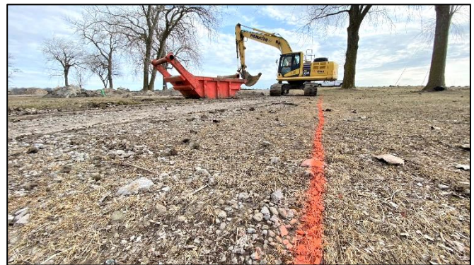
Installation of 8-inch water main at Bay Point, 3/6/2023. The orange line indicates the planned alignment.
