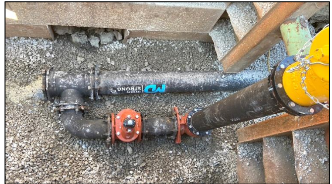
Installation of 8-inch water main at Bay Point, 3/20/2023.
