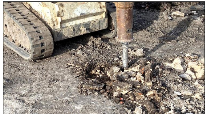
The playground contractor using jackhammer to excavate for the footers, 4/10/23
