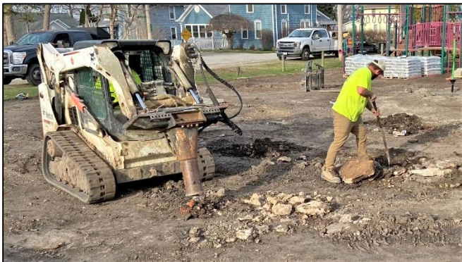
The playground contractor using jackhammer to excavate for the footers, 4/10/23
