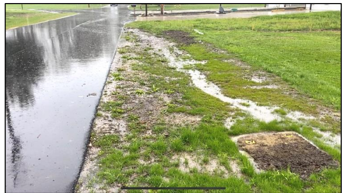
Heavy rainfall on 4/28/2023 showing effectiveness of grading adjustments to improve drainage on Elliott St.
