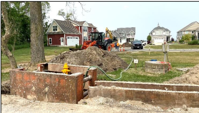
Installing the 8-inch watermain loop to link the existing dead-ends
