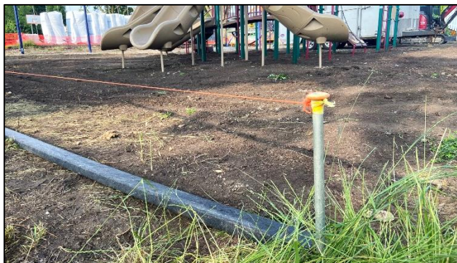
The first step in the turf installation was to adjust and set the site grading
