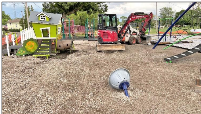
Tilted spinner seat damaged during turf installation
