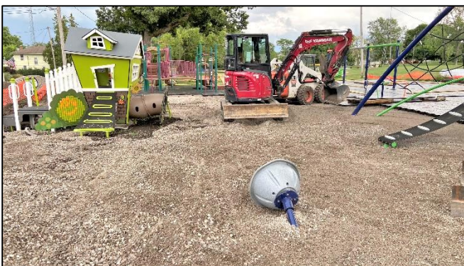
Tilted spinner seat damaged during turf installation
