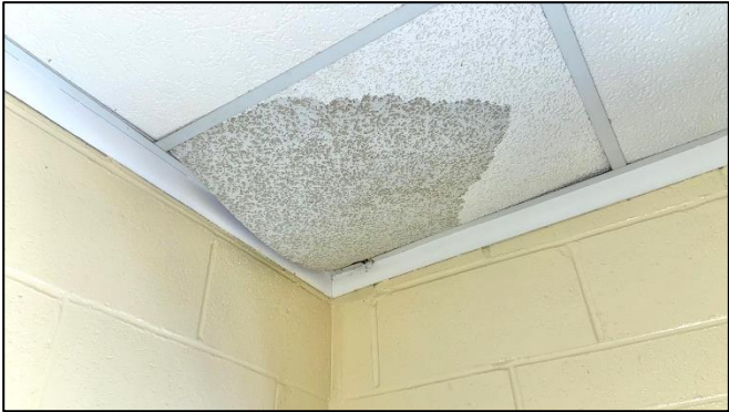
Evidence of a roof leak at the water plant
