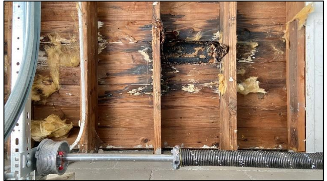
More leaks in the garage roof
