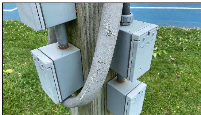
Deteriorated wiring on the auxiliary pole
