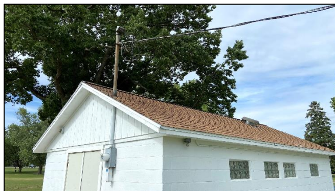
Overhead electrical service to the restroom building
