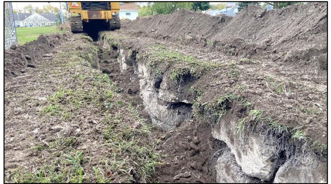
Gill Construction excavated the trench, which revealed how close bedrock is to the ground surface.
