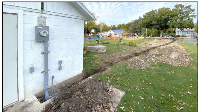
A.T. Emmett installed the electrical conduit and mounted the new meter.
