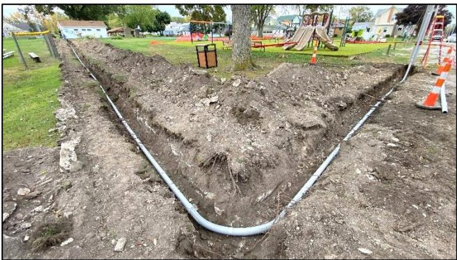
A.T. Emmett installed the electrical conduit and mounted the new meter.
