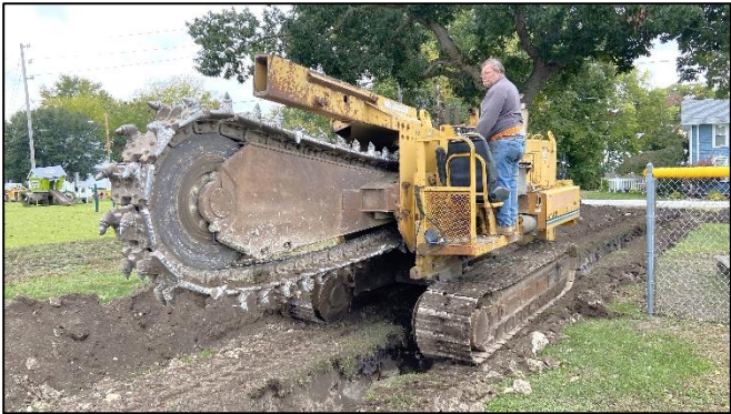
Gill Construction excavated the trench, which revealed how close bedrock is to the ground surface.
