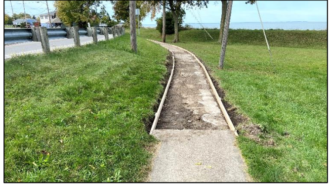
At the Main Street curve, the old sidewalk has been removed and forms installed ready for concrete, 10/23.
