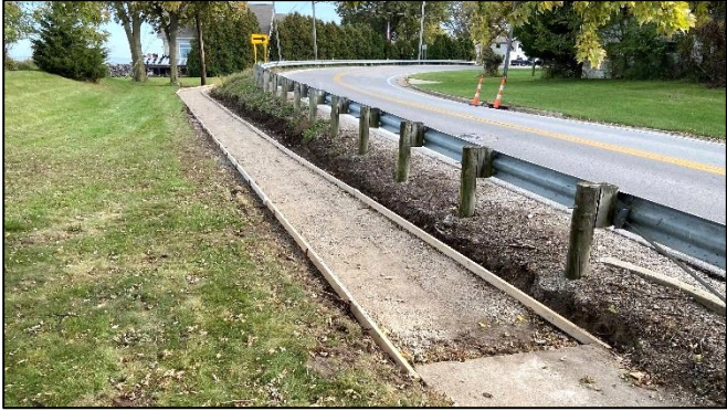
At the Main Street curve, the old sidewalk has been removed and forms installed ready for concrete, 10/23.
