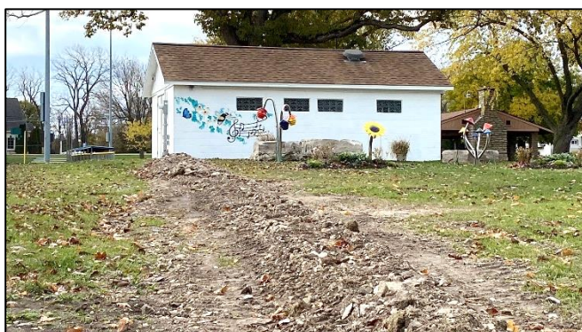
The backfilled trench will be given time to settle
