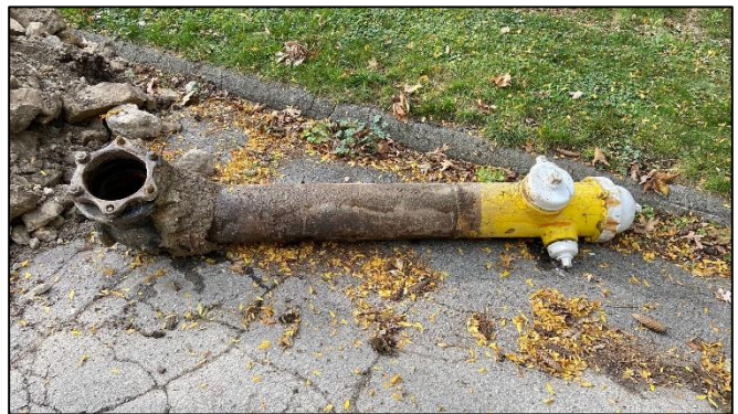
The old hydrant, removed
