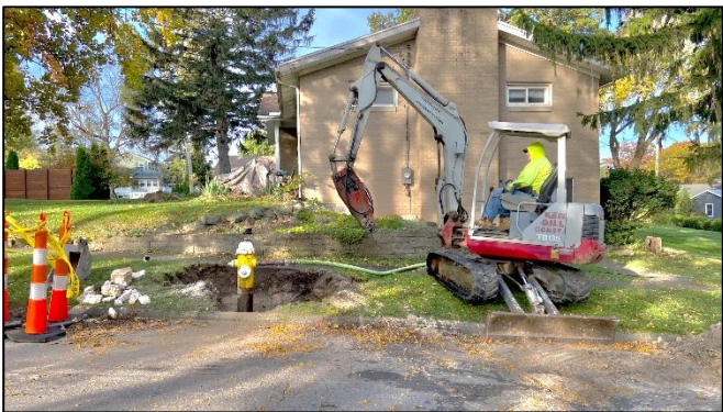
Jack hammer used for busting the concrete
