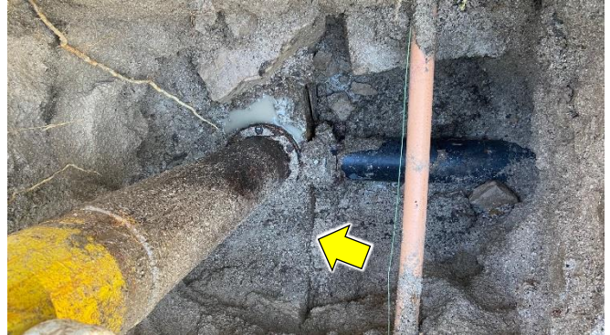
Hydrant's base encased in concrete, surrounded by bedrock
