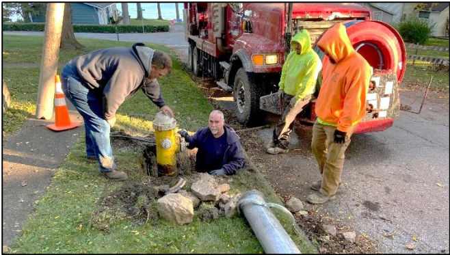
Hydro-excavation to minimize the area of disturbance
