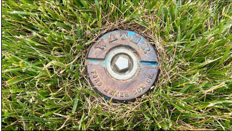
Example of a curb stop cover at the ground surface
